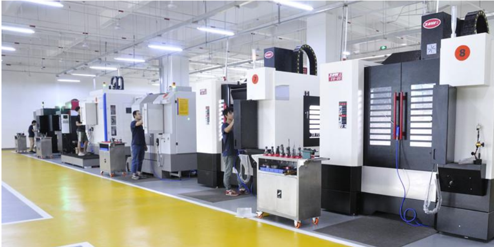
Industrial Oil Chiller Application
